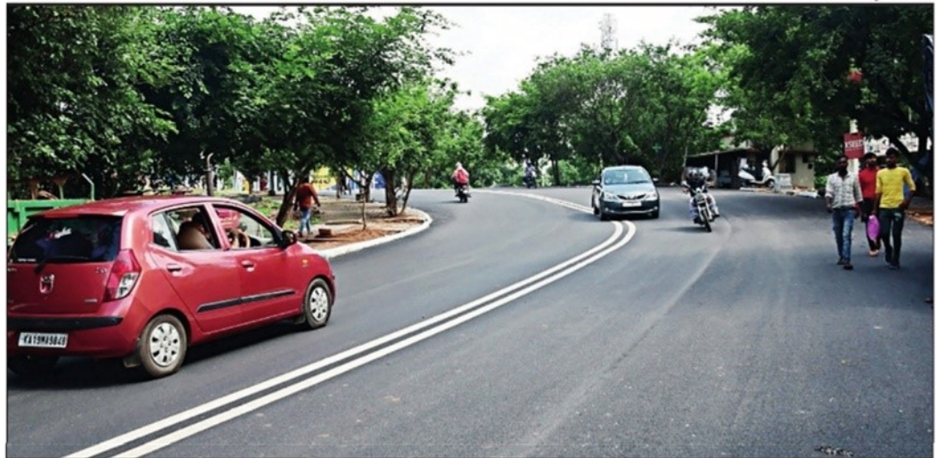
SWANKY LOOK: Apart from the road linking Kommaghatta and Kengeri being asphalted, drains with broken slabs have been repaired and replaced and the whole stretch given a clean look
