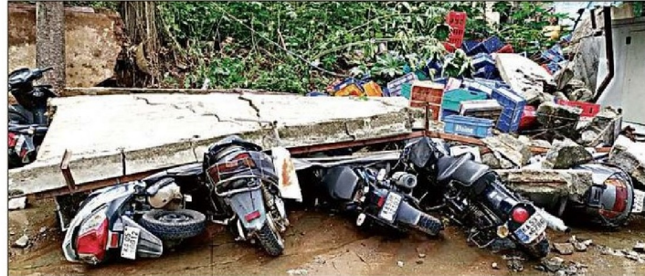
The compound wall of Krishna Theatre in KR Puram collapsed crushing seven to eight bikes that were parked alongside. PHOTO: RAIMA BHAUMIK
