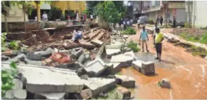
A wall damaged in Singapura Layout as the Singapura Lake overflowed due to heavy rain on Friday night | ASHISHKRISHNA HP
