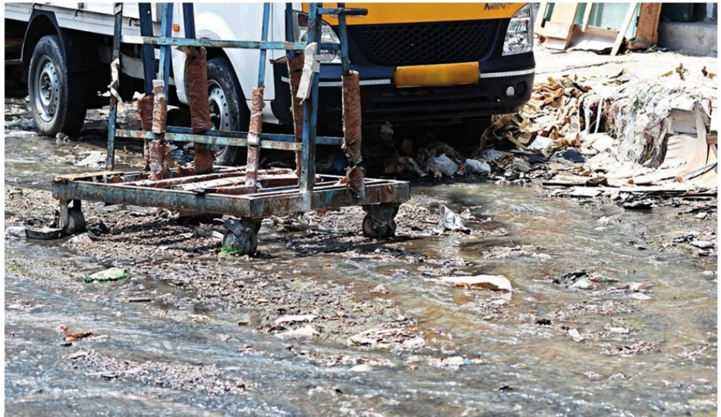
Sewage gushes out of manholes and floods the streets soon after a short spell of rain in some areas
