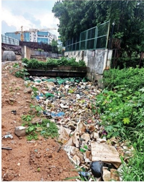
Debris blocks Rajakaluve near Marathahalli
